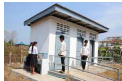
The project engaged teachers, students, parents and local authorities to build three blocks of latrines in the primary school in Ta Nang village. Older students teach their younger peers how to use it and how to wash their hand afterwards. "Open defecation makes areas around our school dirty and smelly. The latrines are very easy to use and we feel safe using it, no rush," says 14-year old Bao in grade four.
